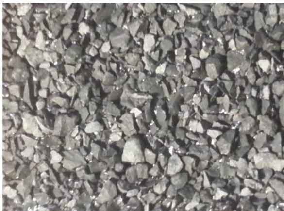
**Before sealing:** with air spaces between the shingle's protective granules. This slows moisture loss, helps moss get established, and as water freezes between the granules, can pop them off.
